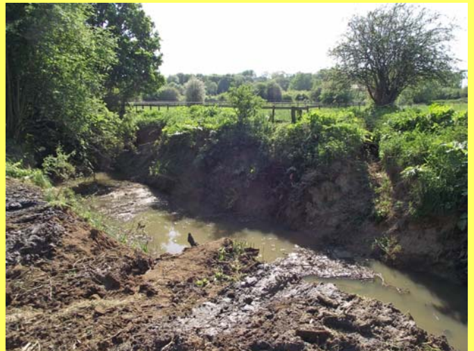
After clearance: "A good day's work"
