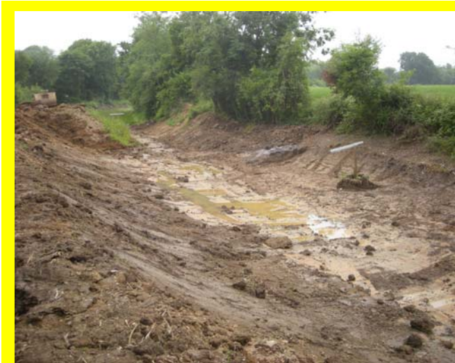
The result of the recent reprofiling at the Devil's Hole Pound (Geoff Thomas)
