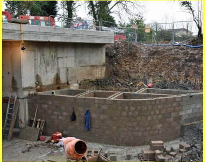
**Compasses Bridge - the south western wing wall. The concrete blocks form the shuttering for the structure which will be filled with concrete. The outside surface will be clad with facing bricks. (Photo: Dave Verrall)**
