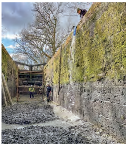
Repointing at Baldwin's Knob Lock
