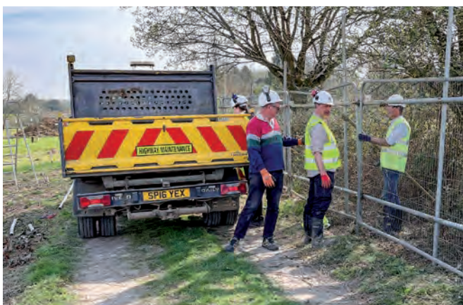
Erecting tree protection, required before work can start
