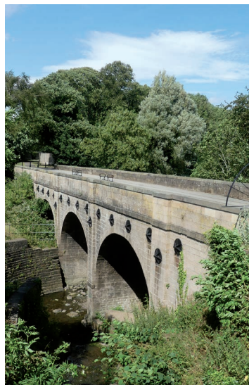
Jessop's Kings Mill Viaduct, Mansfield
