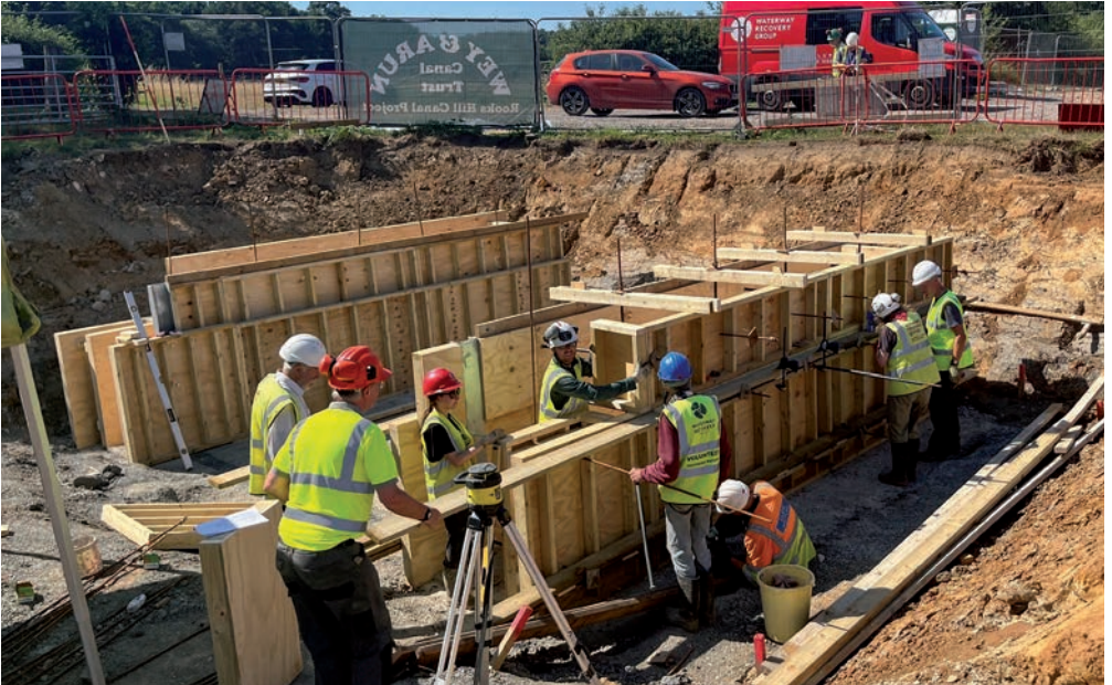
Above: July 8th - Rapid abutment formwork progress by the WRG Below: July 17th – just 32 days from digging the first sod, the bridge abutments are revealed
