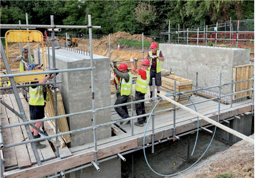
Above: July 8th - Rapid abutment formwork progress by the WRG Below: July 17th – just 32 days from digging the first sod, the bridge abutments are revealed
