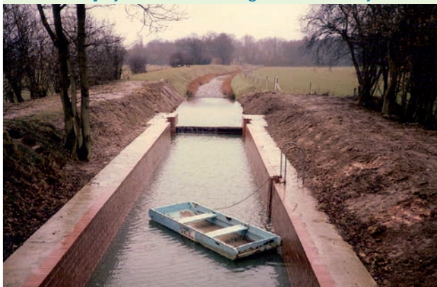
Rowly Lock (Lock 17) and bridge - sadly not currently accessible.
