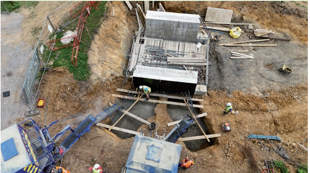
Aug 18th: The base of the first two wing walls are poured. Two trucks pour concrete simultaneously to avoid the clay wall between the two slabs collapsing. Clever thinking by our EWG team!
