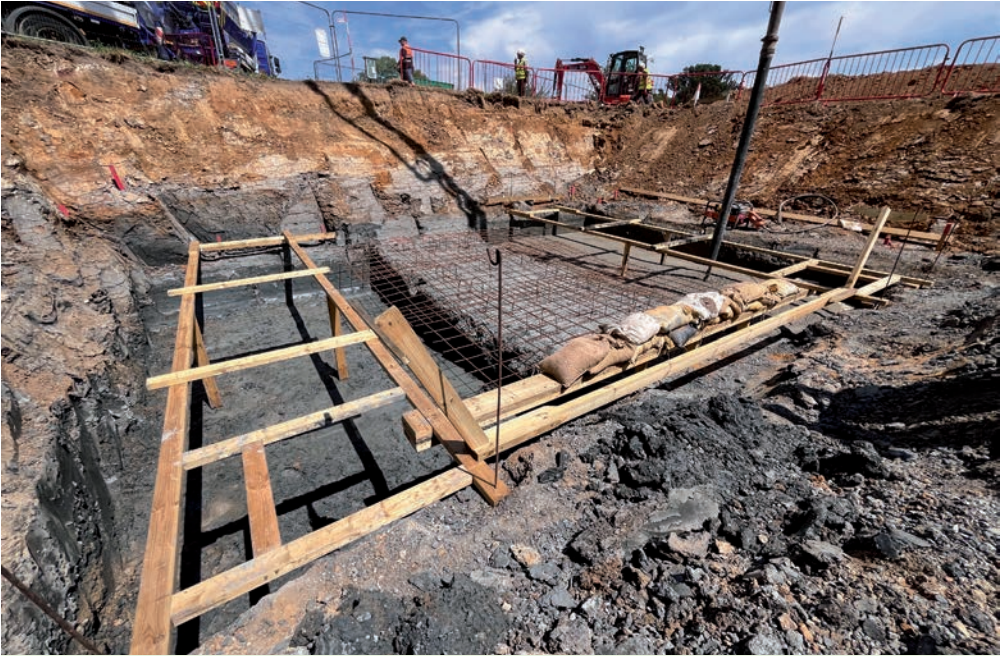
Above: July 1st - Day 16 - Laying the bridge foundations. Below: Waterway Recovery Group (WRG) volunteers beginning the formwork.
