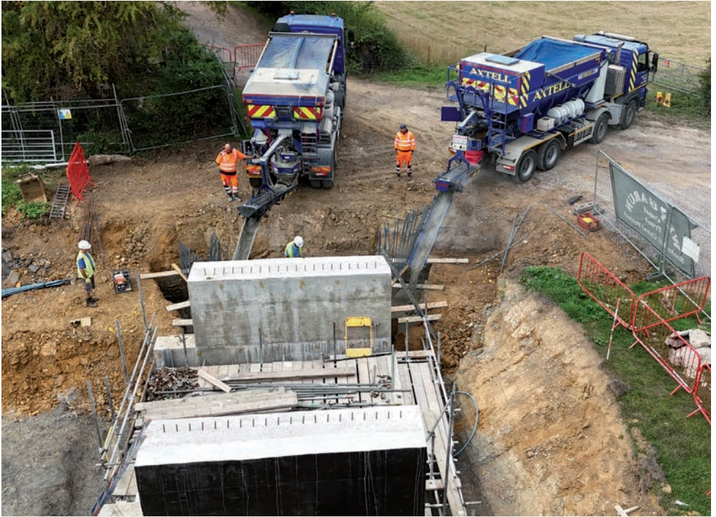
Aug 18th: The base of the first two wing walls are poured. Two trucks pour concrete simultaneously to avoid the clay wall between the two slabs collapsing. Clever thinking by our EWG team!
