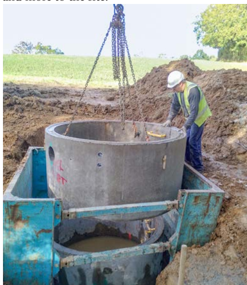
The top ring being guided into place by Pete Turville (NWPG)
