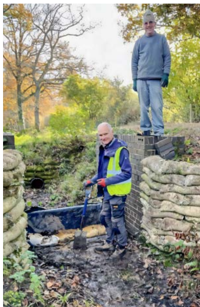
Fitting temporary stop weirs
