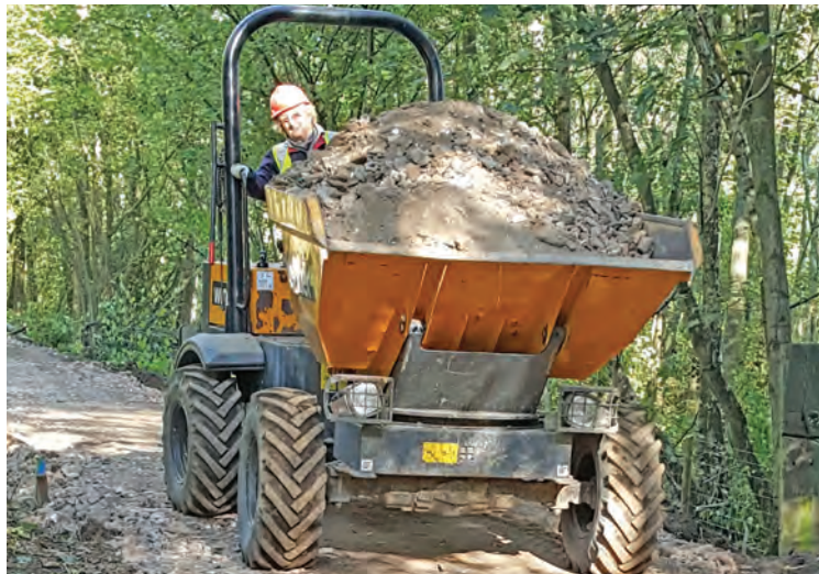
Driving on: work at Birtley Reach gets under way
