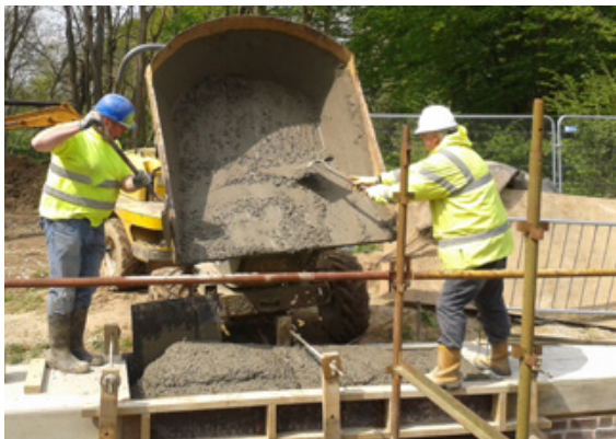
Pouring concrete for the copings at Gennets Bridge Lock. (Geoff Thomas)
