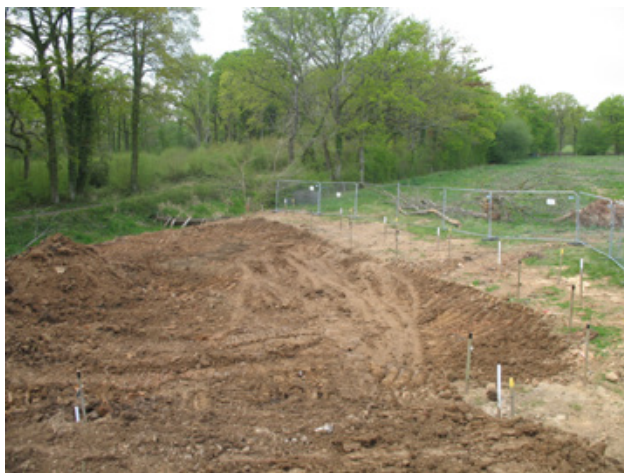
The site of the future Gennets Winding Hole. The white markers show where the fence and hedge will be. The black-topped posts mark where the top of the bank will be. Volunteers are removing the topsoil within this area. (Eric Walker)
