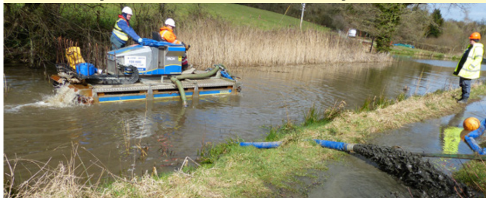
Above: The machine goes to work pumping silt out of the section near Drungewick Lane. Below: Getting to grips with the notoriously shallow Birch Copse section.
