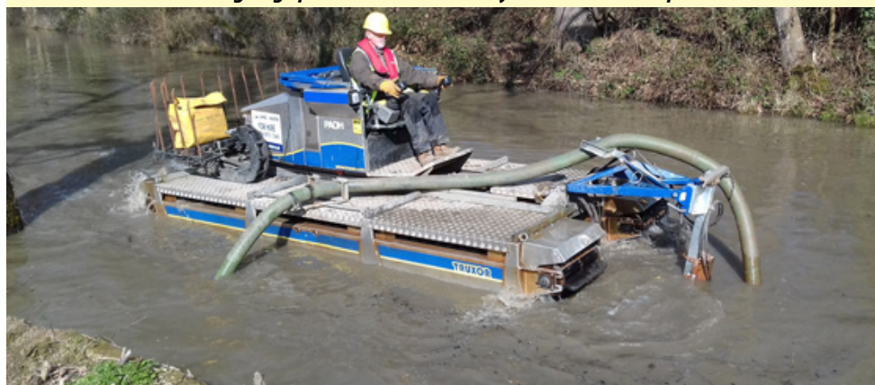
Above: The machine goes to work pumping silt out of the section near Drungewick Lane. Below: Getting to grips with the notoriously shallow Birch Copse section.
