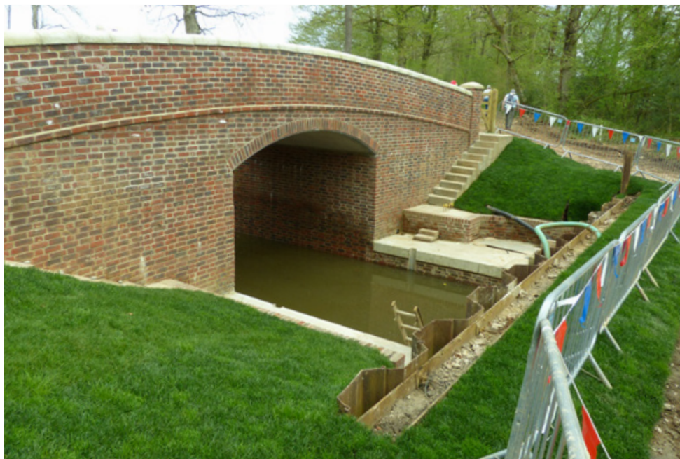
The south end of Gennets Bridge on 21st April. Above: Looking north, showing the new bridge (Geoff Thomas). Below: Looking south from the bridge. (Stephen Batey). The causeway and the piling will be removed as soon as conditions permit.
