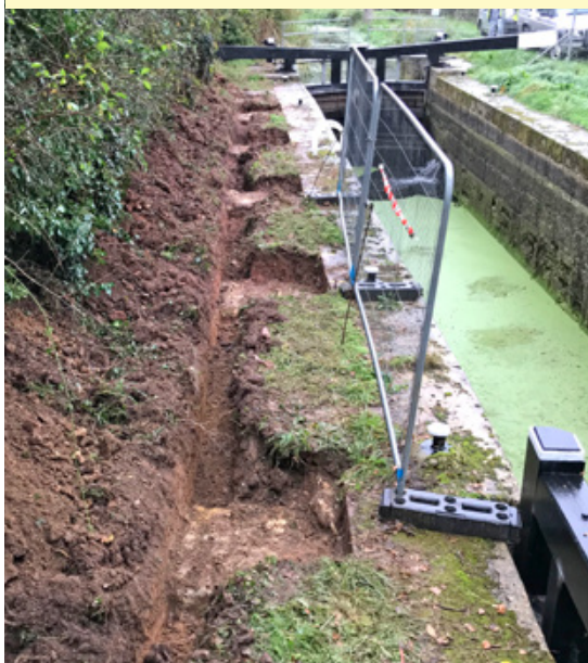
The picture clearly shows the five counterforts uncovered by EWG's investigation.
