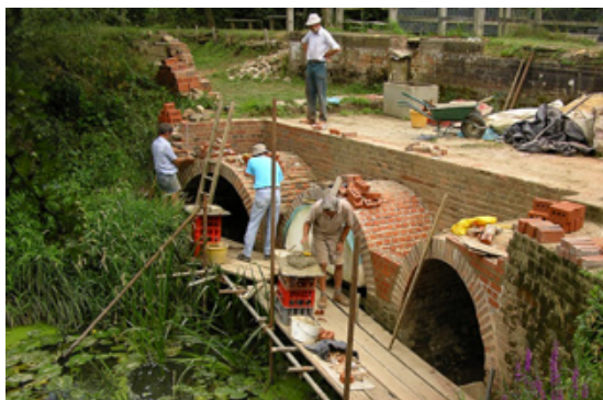
In this archive picture, the Orfold Aqueduct Group volunteers are widening the brick arches at the Aqueduct.
