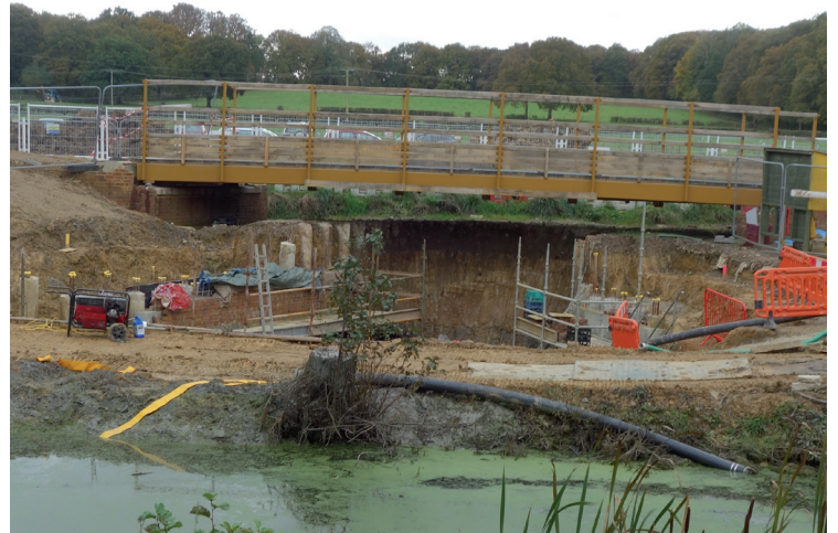
Progress at Tickner's Heath near Alfold.
