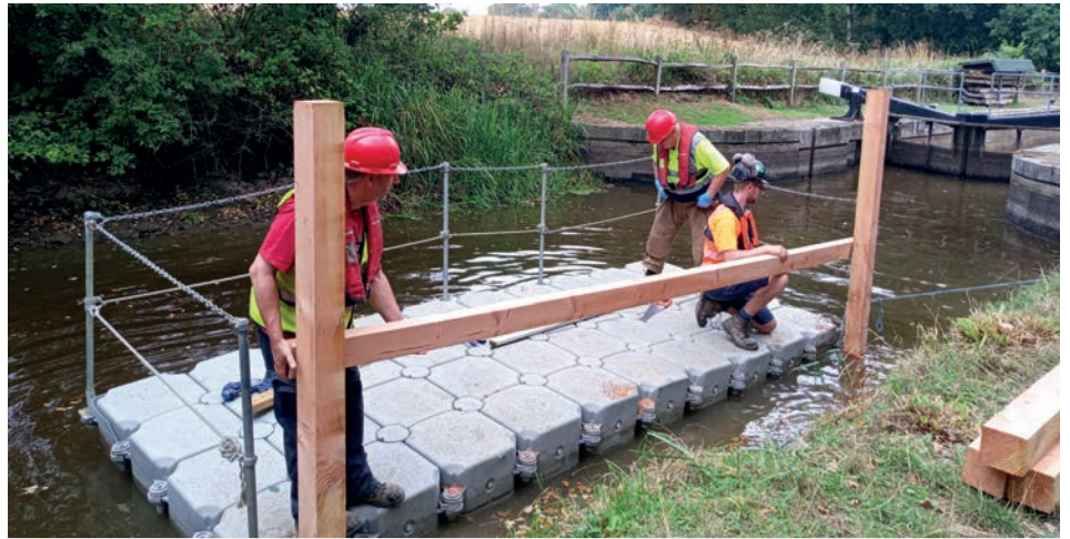
Building a landing stage at Loxwood
