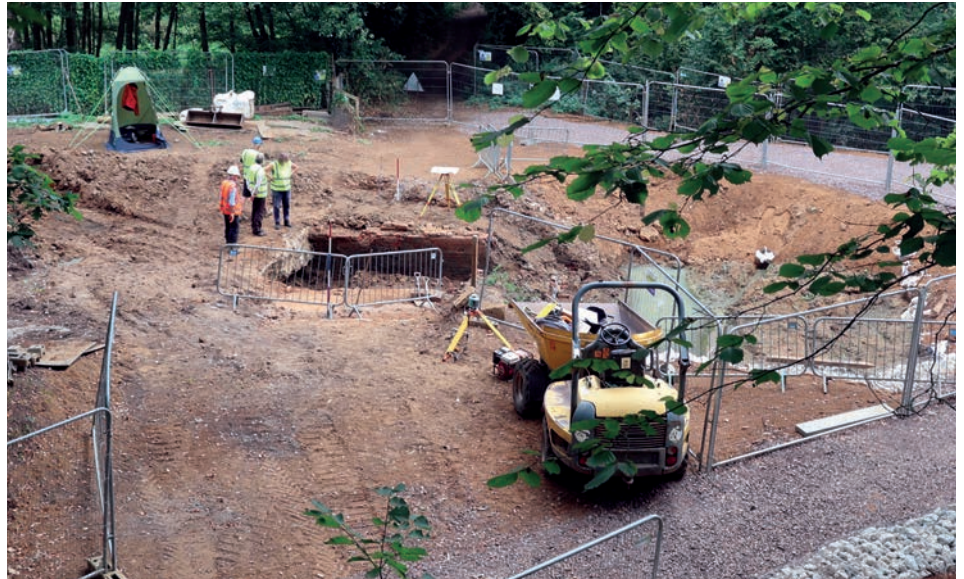
Excavation at the original bridge (centre) and the diverted bridleway (right)
