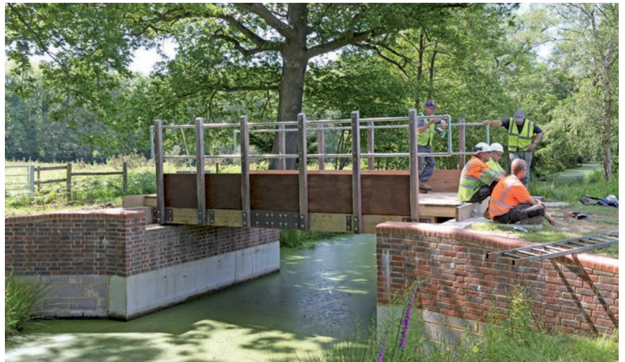
The first of two bridges that will soon have lifting decks
