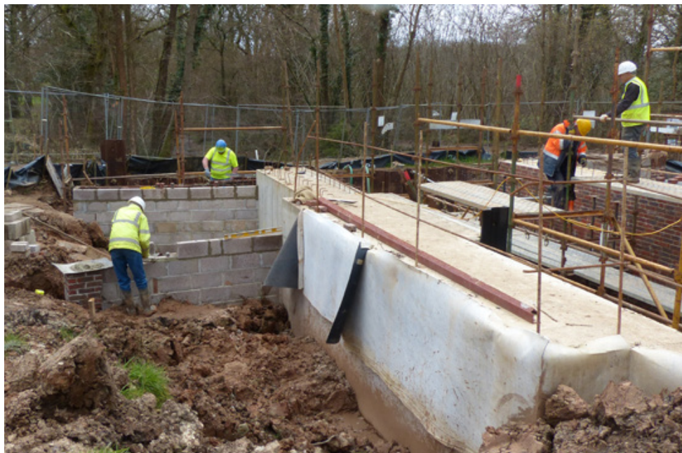
Putting the “Bridge” into Gennets Bridge Lock. Top: the deck of the new bridge is on the right. Below: a first view of the bridge arch from inside the lock.
