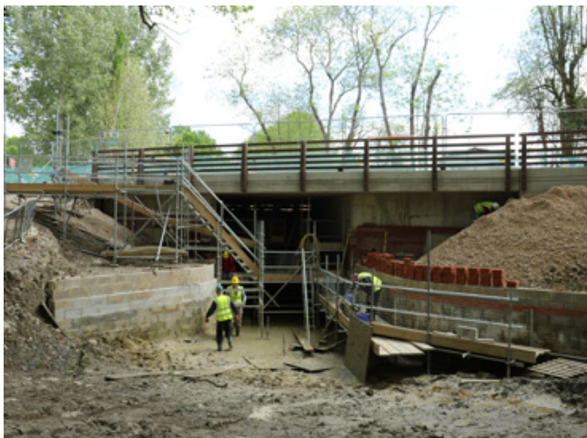
A mid-May view of the south side of Compasses Bridge shows progress with the brick facing.
