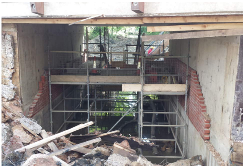
Above: Breakthrough! On 14th May the WACT digger equipped with a powerful 'pecker' removed the old causeway wall at Compasses Bridge. (Peter Jewell) Below: The Trust's Mobile Display Vehicle is on the road again and seen here at the Merrist Wood College Summer Show on 15th May. (Julian Nowell)
