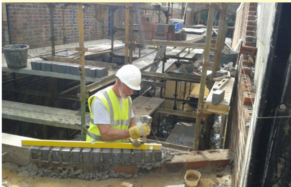
Above: Geoff Thomas lays the last brick for the walls of Gennets Bridge Lock. Below: Edward Stratton-Woodward laying bricks along the curved wall at the top cill of the lock. (Pictures by Geoff Thomas/Len Hasler).
