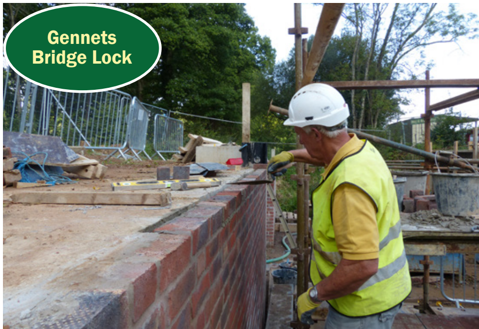
Above: Geoff Thomas lays the last brick for the walls of Gennets Bridge Lock. Below: Edward Stratton-Woodward laying bricks along the curved wall at the top cill of the lock. (Pictures by Geoff Thomas/Len Hasler).
