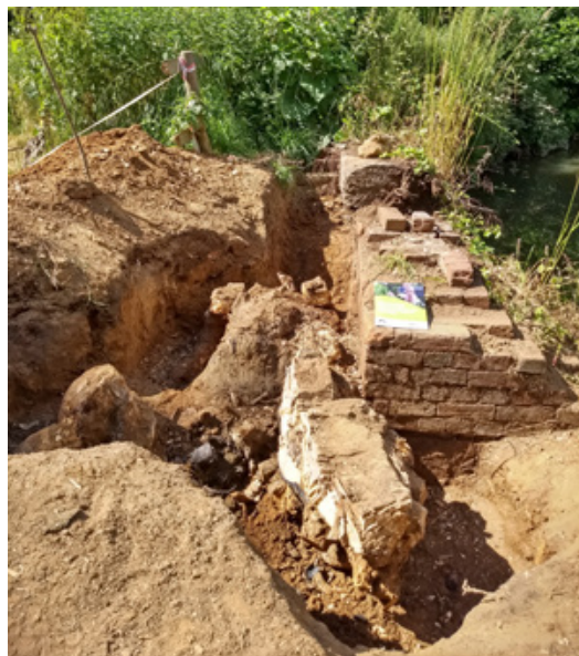
The tree root at Gosden Aqueduct that stubbornly resisted all attempts at removal until tackled with a stump grinder. (Nick Houston)
