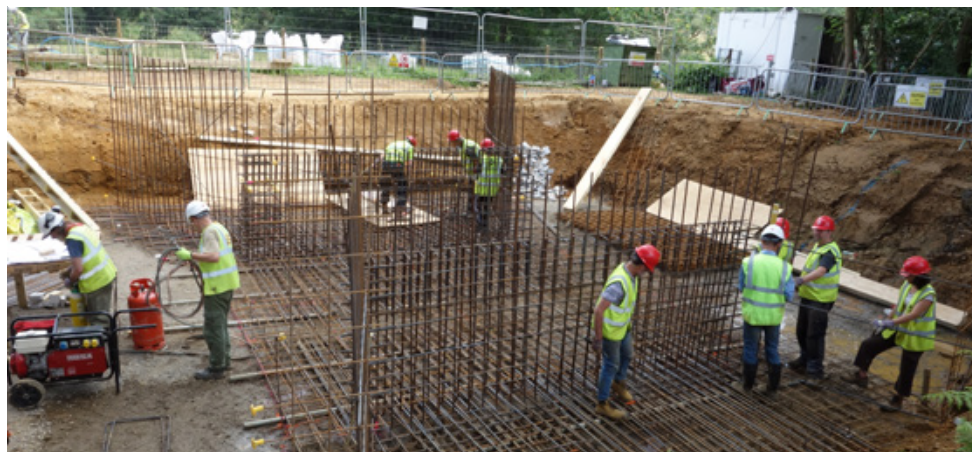
The steel frame came together in time for a concrete pour at the end of the week.
