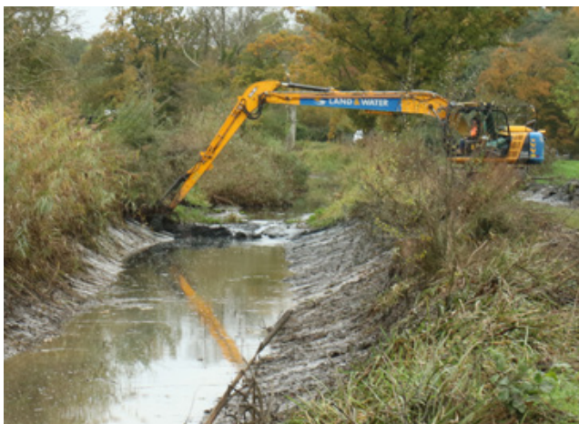
Top: The Aquamaintain team repatriated more than 8,000 fish in a half-mile section. Above: Land & Water are desilting before the leaks are plugged.
