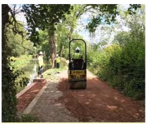
Clockwise from top: Dave Evans prepared the areas to be resurfaced using the digger, which just managed to fit along the towpath; volunteers then covered the holes with hardcore and limestone scalpings; the final stage was to roll the material flat to create a smooth path.
