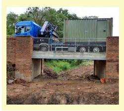
Volunteers reprofiled the area around the new bridge, completing the gradients on both sides of the bridge along with the ramps. The next step was to remove the temporary bridleway diversion created at the start of the project. The result is a much improved path for walkers, riders and cyclists.
