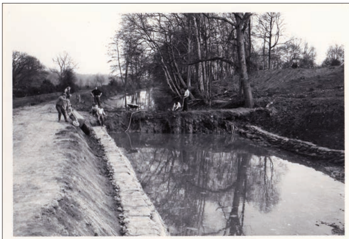
Left: Volunteers installing bagwork to secure the repaired canal bank at Birtley, circa 1976.
