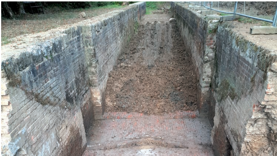
Clearing the lower entrance and gate recess revealed damage to both north and south walls.
