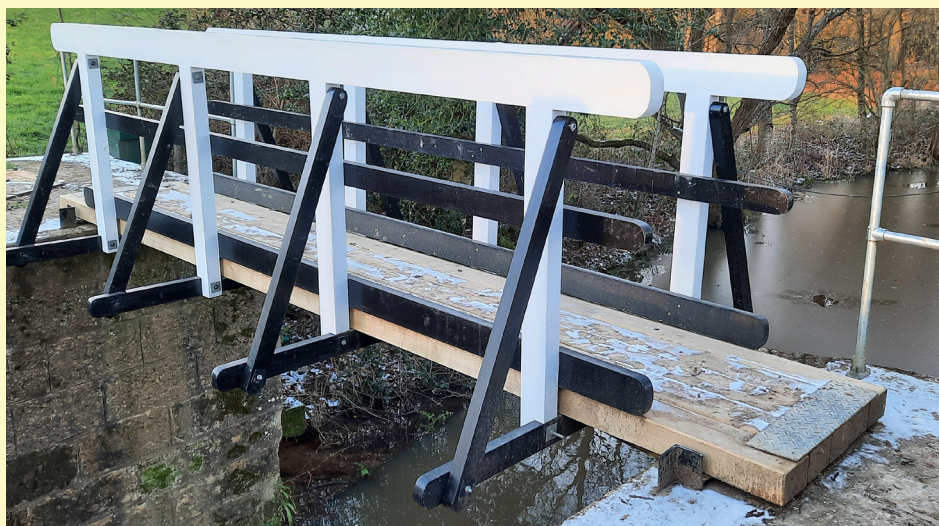
The replacement footbridge at Baldwin's Knob Lock is now in place. The Tickner's Depot team began fabricating the bridge last year but lockdown prevented them finishing the job. Kevin Baker stepped in and he and his team have installed the finished article.
