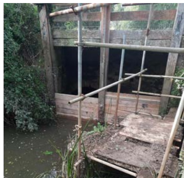
New boards were needed at the weir at Lordings waterwheel.
