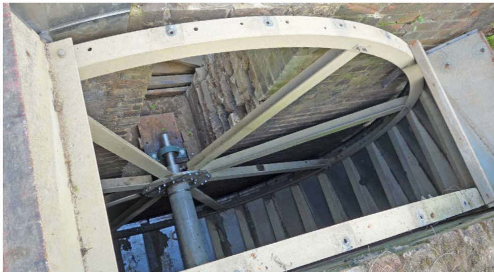
A specially designed stainless steel shaft was commissioned, and a replacement chute fitted.
