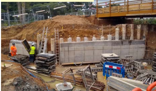
The training walls taking shape at Tickner's Heath.
