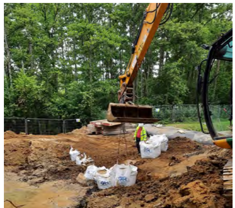
The temporary bridleway under construction.
