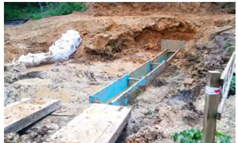
Metal trench boxes were part of the eventual solution.
