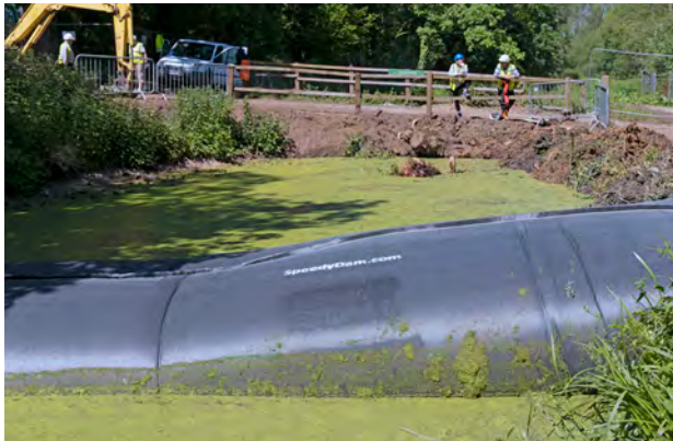
The SpeedyDam installed across the canal. (Bridge 2 site in the background).
