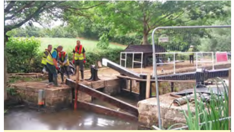
By the end of June we could remove the stop planks and put the lock back into water.
