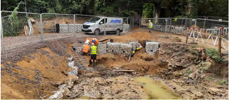
Gabions and Platipus anchors provide stability to the west bank.
