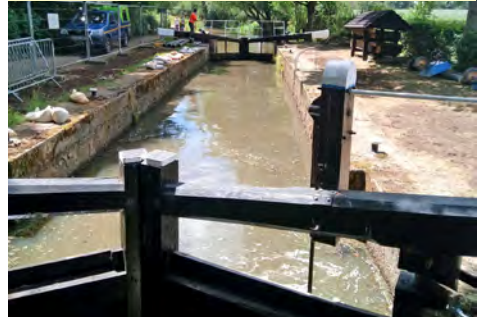
By the end of June we could remove the stop planks and put the lock back into water.
