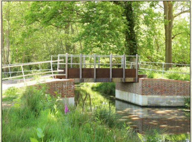
Birtley Bridge 1, near Bramley (Surrey), built by volunteers on a section of canal newly acquired by the Canal Trust
