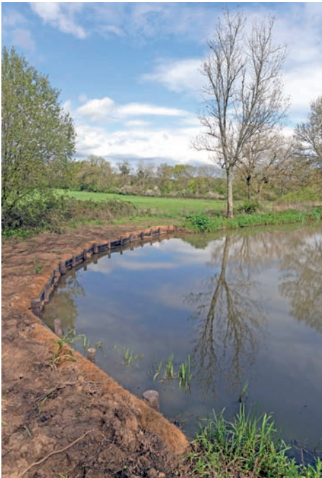
Completed work at Brewhurst Winding Hole
