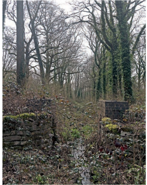
The site of Lock 11
