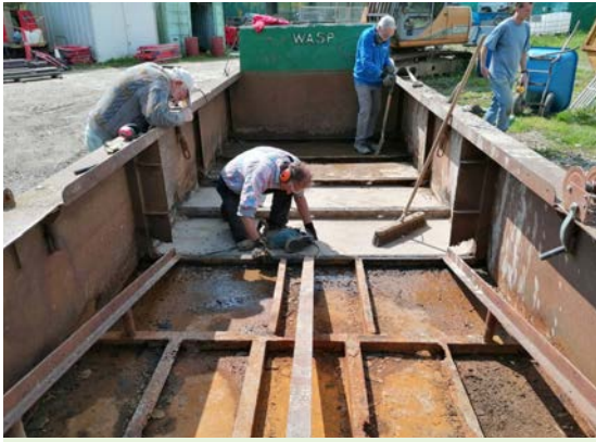
Repairing ‘Wasp’ - a slow process
