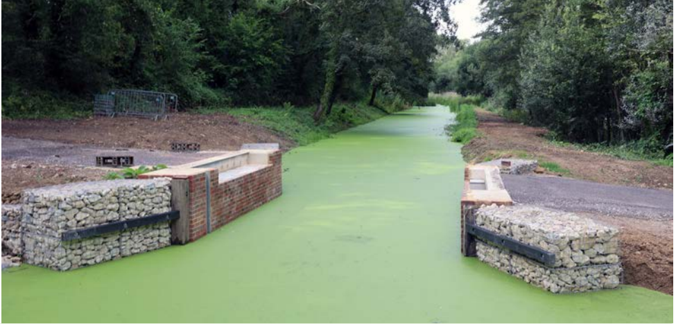
Bridge No 2 – today's finished abutments (above)
