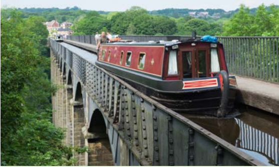
The Pontcysyllte aqueduct on the Llangollen Canal
