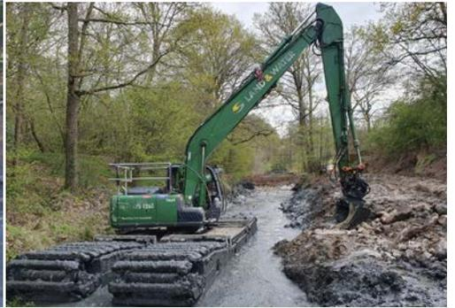
*Desilting in progress with the contractor's dragline (left) and amphibious long reach excavator (right)
