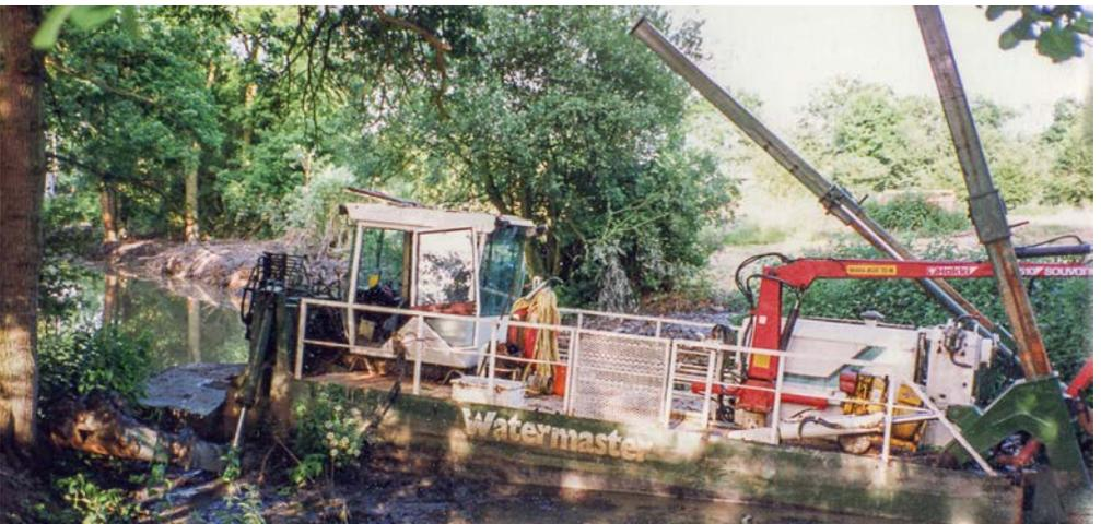
*Initial desilting in the 1990s using a hired-in Watermaster machine*
