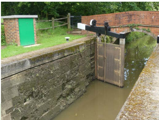
One of the new cabinets - here at Devil's Hole Lock
