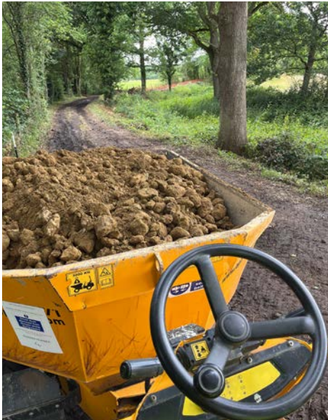
Base stone ready for laying on the old mud
