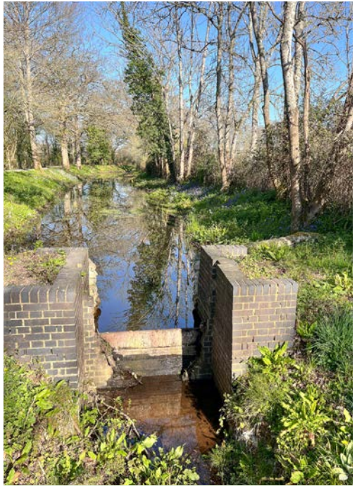
One of the temporary dams north of Gennets Bridge Lock
