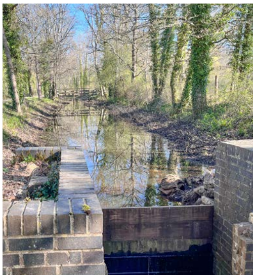
Bonfire Hanger and one of the dams
