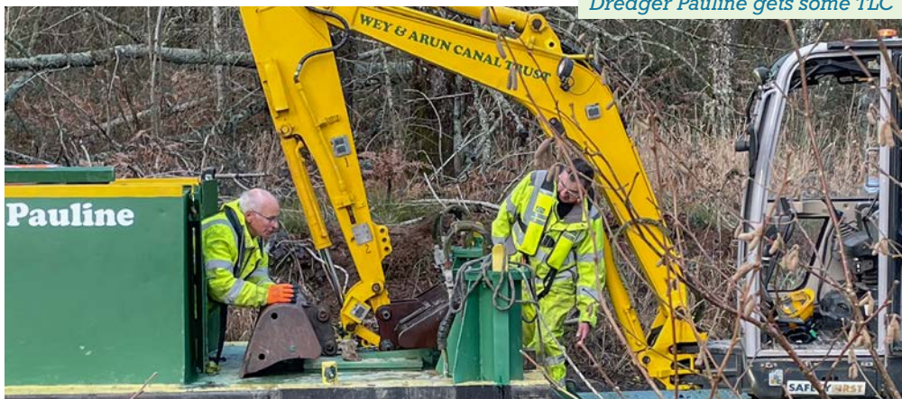
Dredger Pauline gets some TLC
