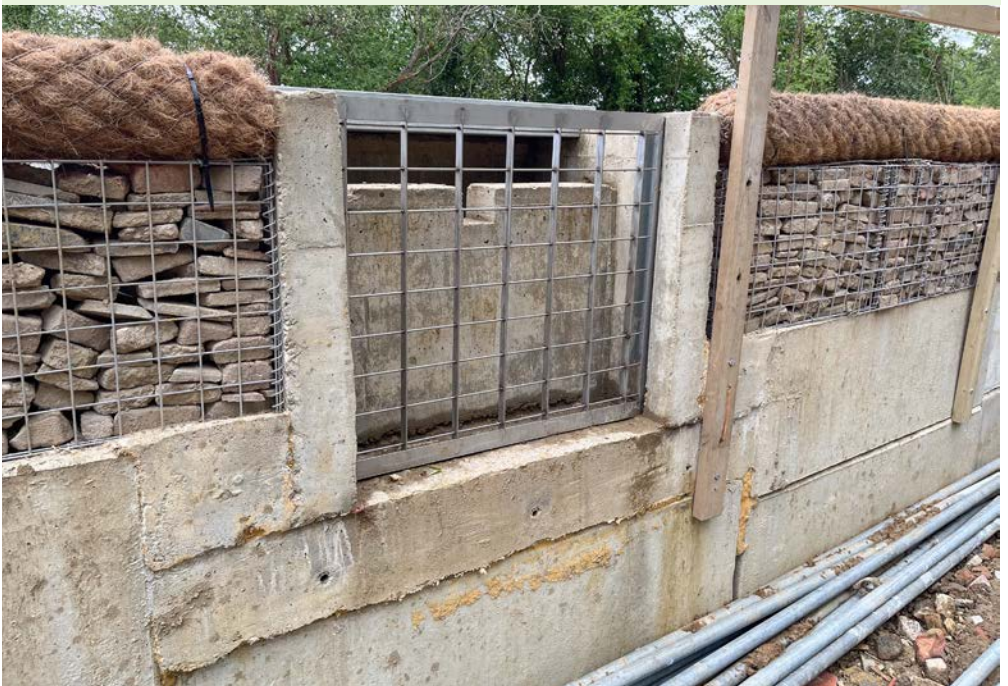
Above : two types of mattresses will hold the western canal bank in place Below : the overflow weir, which will pipe surplus water down to the stream
