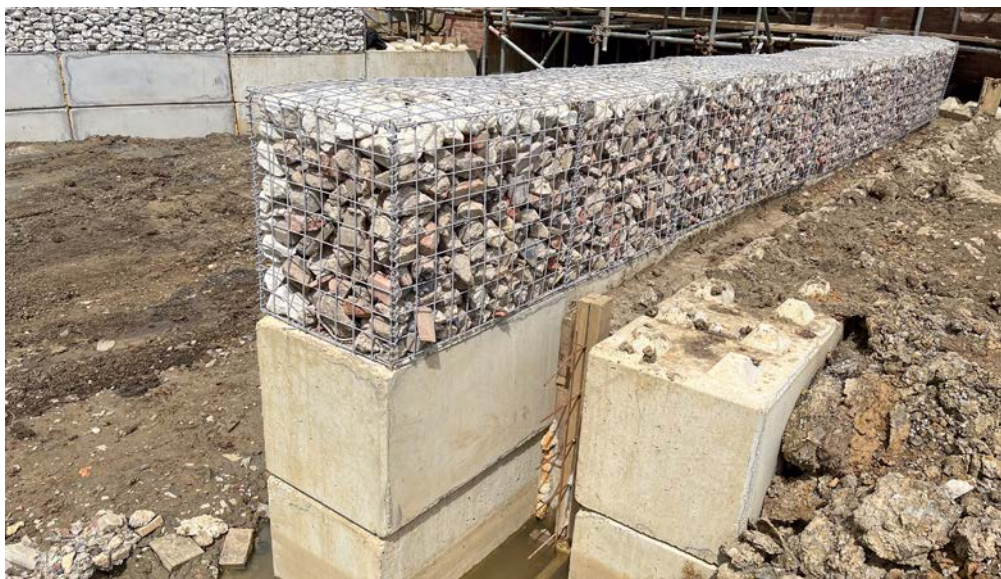
Interlocking concrete blocks and gabions in the wall leading to the new bridge
