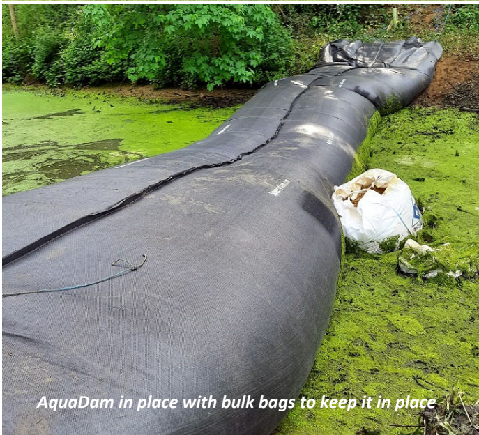
Installing the AquaDam
