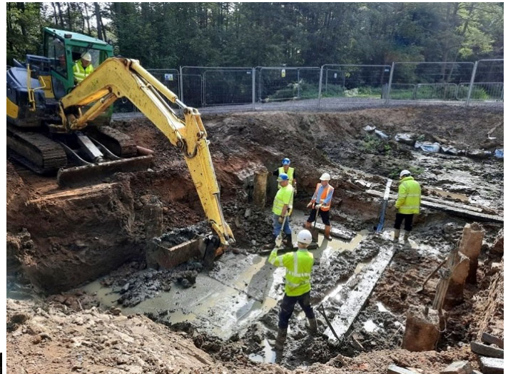
The piles installed and a start being made on the concrete blinding
