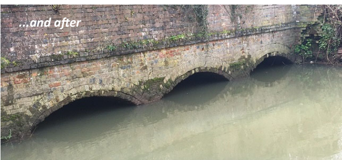
Gosden Aqueduct before...
