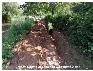
A pedestrian trencher was then hired, with much less soil being removed during the digging process which in turn meant there was considerably less backfilling to be done!
