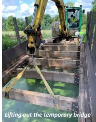
well embedded screw/bolt fixings. Then, we managed, with a method suggested by Dave Evans, to remove the heavy timber and steel deck framework in one go using our Yanmar digger.
