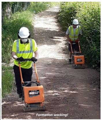
For the remainder of the month, work continued on reinstating the towpath with much surface dressing and wacking! The towpath was subsequently reopened for public access.
