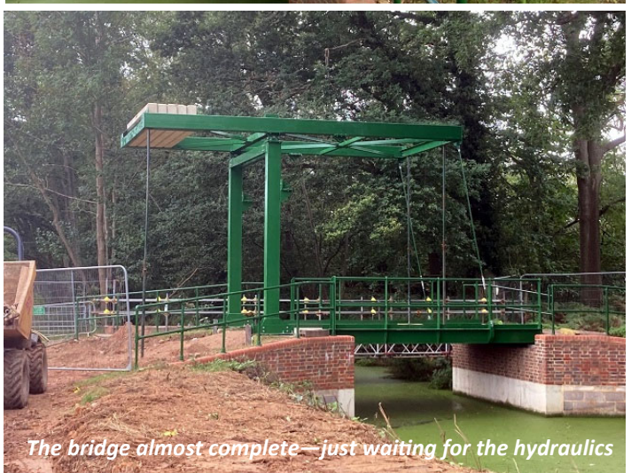
Construction at Birtley Bridge 1
