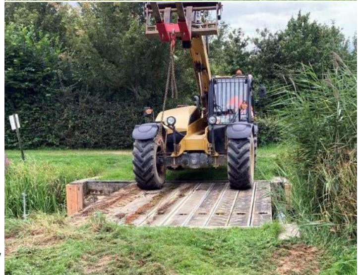
Installing the Heavy Plant Crossing
