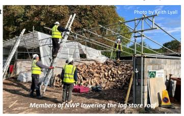
Longitudinal poles were removed, with the Ledgers, and repositioned 60cm lower. The guys did an excellent job and finished the first of the three bays. Two days later the left bay was also lowered. The roof materials have now been delivered and I can see this mini project will be ready for a topping out ceremony in the very near future.
