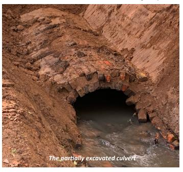
hole four metres square and five metres deep. After excavating to expose the culvert we decided to remove the whole top section and lay double wall plastic pipes 25m long into the total length of the remaining brick lower section.
