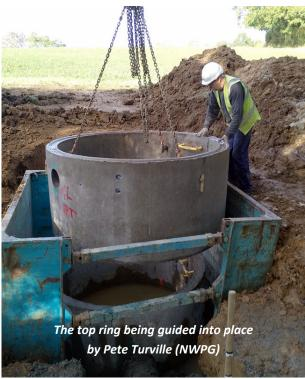
ring was then lowered in and concreted into place; the difficult task being the lining up of the connecting pipes to and from the dragon's mouth.
