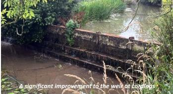
A little further down the canal toward Lordings Flood Lock is a small spill weir, where there was concern about water leaking from the canal around the structure. We excavated a small trench on either side of the weir and packed it with puddling clay, that again had been kindly donated by Ewhurst Brickworks. The water level is so low in that section, at the moment, that we are unable to assess the effectiveness of our
