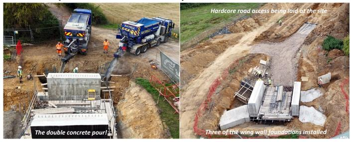
While the weather has been kind, we've been planning ahead for when the rain inevitably makes the site a bit soggy. So we've been laying a hardcore access road across the site and along the bed of the canal over the clay strata. Otherwise any movement of plant or vehicle deliveries would be precluded when the weather turns wet.
