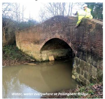
We had planned to complete filling the towpath wall and for our specialist contractor to install the four Cintec anchors to the stone bridge foundation walls on the 16th December, but when the team turned up that morning there was a good metre of flowing water going under the bridge and all work had to be aborted.
