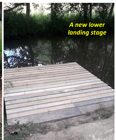
Completed repairs at Baldwin's Knob
