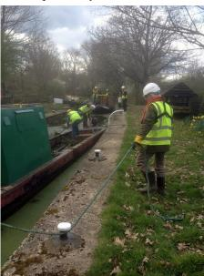
Initially the team cleared debris from the water and cut back vegetation on the offside down to BKL. Subsequently the team went up to DHL again clearing the banks to the extent allowed at this time of year and removing debris and floating vegetation from the water.
