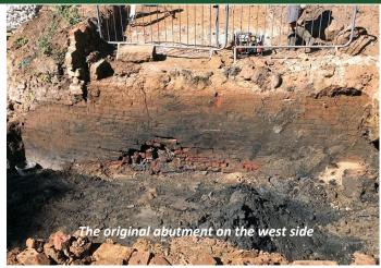
of the brickwork was supported by timbers 4" thick and 12" wide for the full width of the wall and run-
