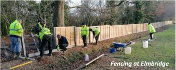
140 four feet high wooden panels, with concrete posts and gravel boards, are to be installed on a 250 metre section of land that borders the Canal to the south of Elmbridge Road.
