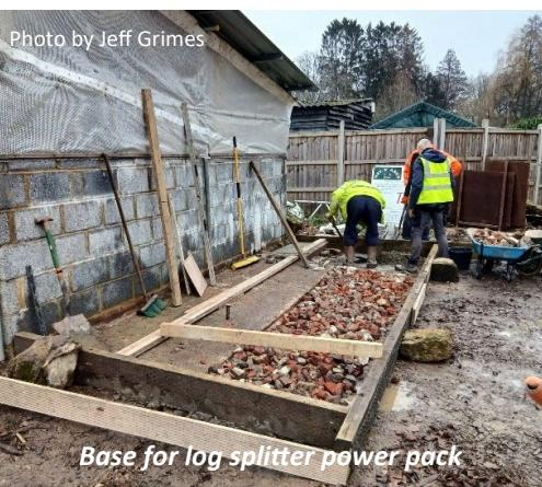
Additionally, our Monday Team has completed a miscellany of tasks with Andy Evans having now completed the build of a custom made diesel power pack for the hydraulic log splitter, they have commenced the preparation of a permanent hard standing for the unit, adjacent to the log bay at Tickner's Depot.
