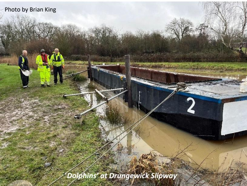
During the month, several visits were made to Drungewick Slipway where we finished constructing and installing two sets of 'dolphins' alongside which the two dredger tubs can be moored without getting snagged on the banks. When water levels permit, another set of 'dolphins' will be installed, so that the dredger can also be securely moored alongside.
