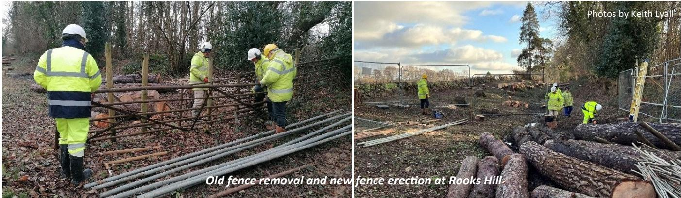
Our attention then turned to the boundary of the canal route beyond the point where the old rusty gates had been. We extended the tree protection fencing a short way along the western bank towards the site of Fanesbridge Lock. Temporary Heras fencing was then installed across the canal route and back along the eastern bank towards the Legato block wall that is already in place by the new weir structure.
