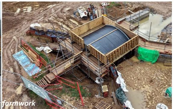
main concrete pour has also been constructed while leaving access for the reinforcing steel to be positioned.
