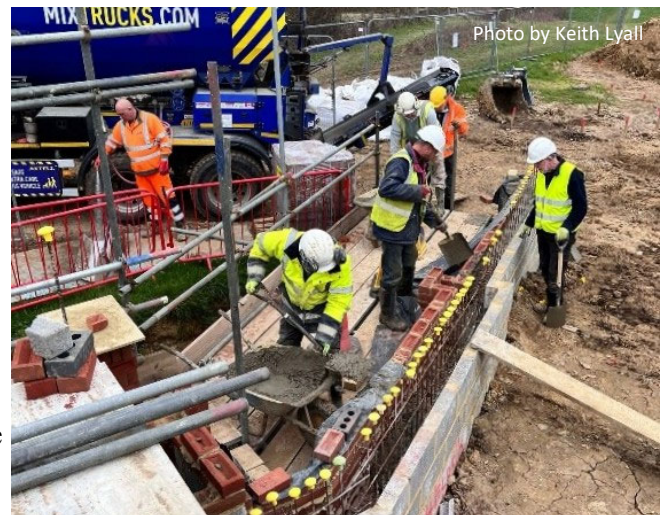
Concreting cavities in wing walls at Rooks Hill Bridge
