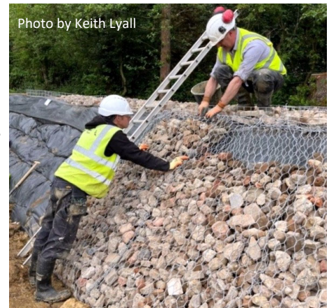
Installing Gabion mattresses
