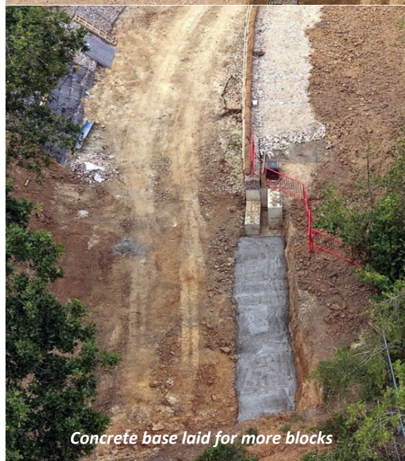
WRG working on the Plastecowood bank for Rooks Hill Phase 2
