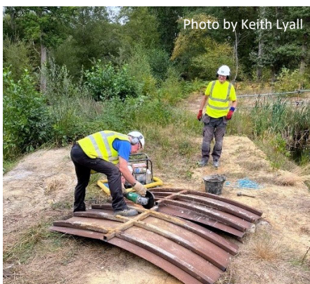
Cutting up the formwork
