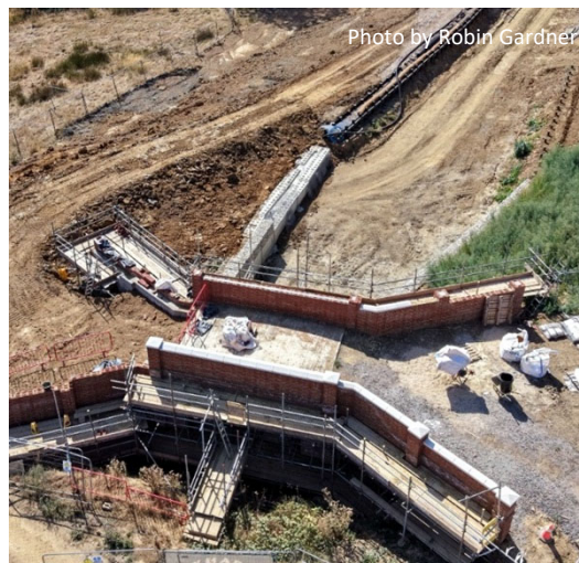
Rooks Hill Bridge with some coping stones
